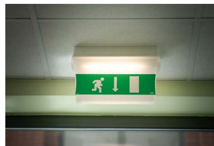
Measurement of emergency and evacuation lighting
